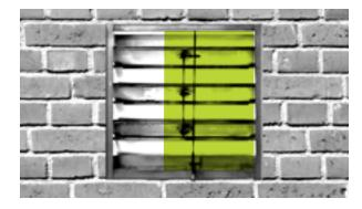
Figure 3: Vent with glass covering 2/3 of vent area
