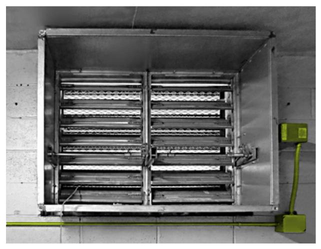
Figure 4: A motorized, fully closing vent
