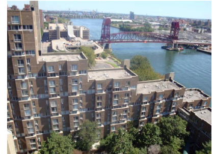
NYC's largest air sealing project
