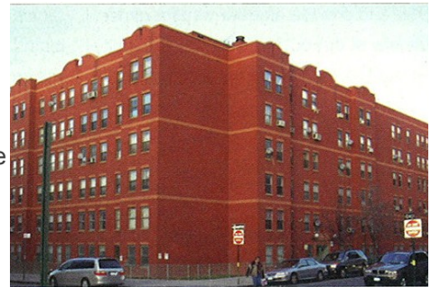
A typical NYC postwar multifamily building with hydronic heat.
