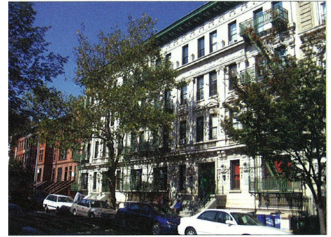
A typical NYC prewar multifamily building with steam heat.
