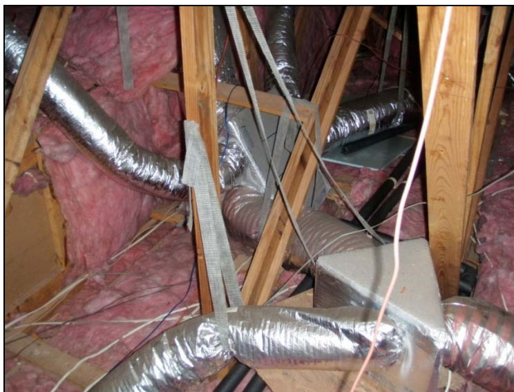
Figure 4. Insulated flex duct in the attic of an existing home
