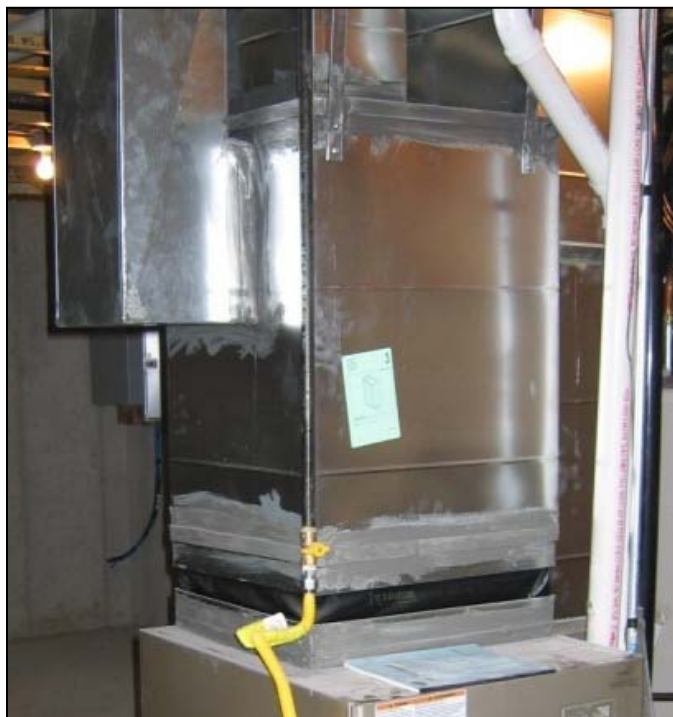
Figure 1. Sheet metal supply plenum sealed with mastic. A flexible, fireproof canvas collar was installed to provide sound/vibration attenuation.
