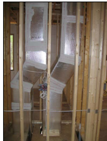
Figure 11. Duct board sealed with mastic.
