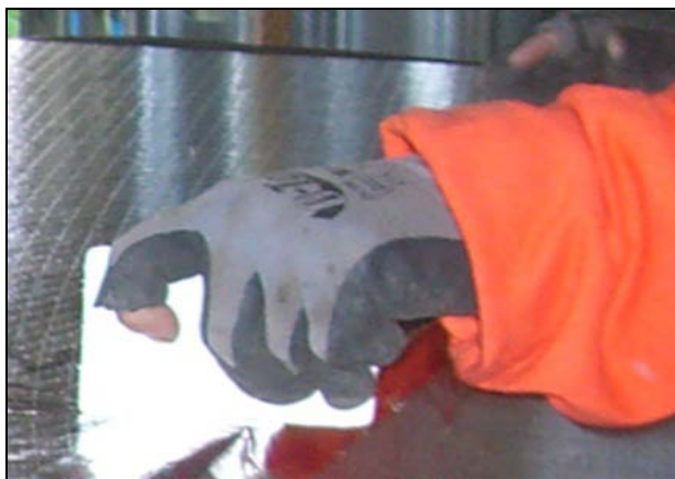
Figure 26. Aluminum tape being smoothed out with a plastic comb
