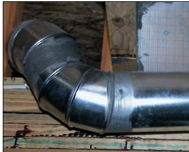
Figure 25. While sealant has been applied to some of these joints, such a thin coat may not provide an adequate seal. Follow manufacturer's instructions for the thickness when applying mastic.
