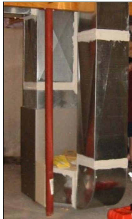
Figure 31. Supply and return plenums and trunks sealed with mastic.
