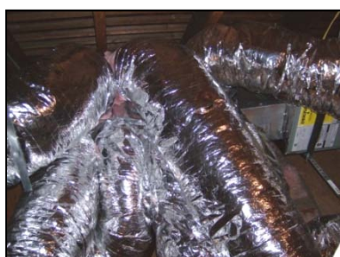
Figure 39. Having this much flex duct branching off at the supply plenum makes it very difficult to properly seal the ducts.
