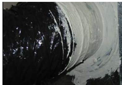
Figure 35 A flex branch (insulation pulled back) attached and sealed to a collar. Note the balancing damper; sealers must be careful that mastic does not prevent access to and operation of such devices.
