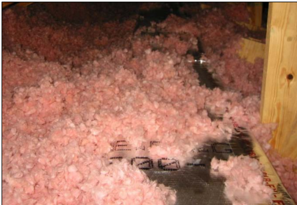
Figure 56. A duct board trunk partially buried beneath blown attic insulation. This may be impractical in existing homes and in humid climates.
