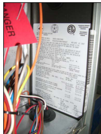
Figure 19. The specified heat rise range for this furnace is 40-70°F according to the faceplate.
