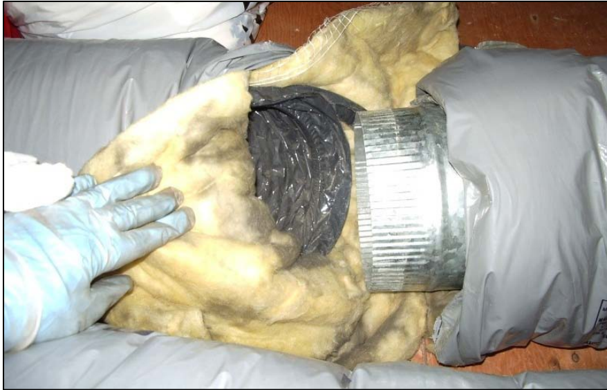
Figure 44. This flex duct junction has failed completely. The inner lining of both sections should be attached and sealed to the metal fitting. Insulation should then be taped in place.
