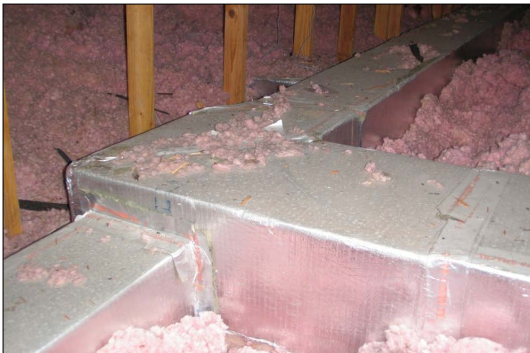
Figure 2. Fiberglass duct board ducts in an attic
