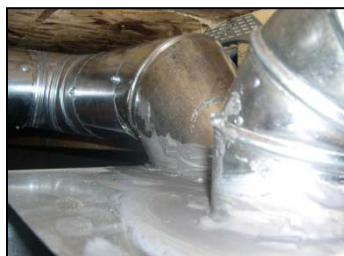
Figure 42. In existing homes, it may be difficult to see all the duct connections, such as these top take-off sheet metal branches. Use of mastic in these tight situations can be much more effective than tape.
