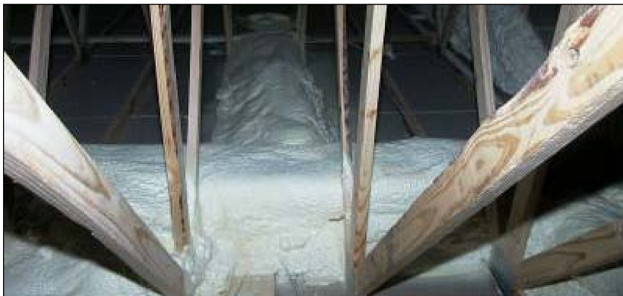
Figure 14. Ducts insulated with closed-cell spray foam in an attic. Fiberglass insulation will be blown over the ducts, providing the necessary ignition barrier.
