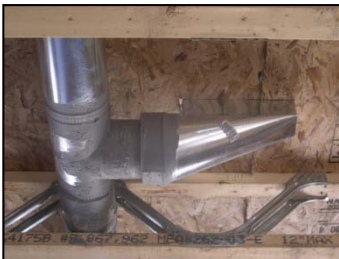
Figure 48. Sheet metal boot that has been sealed.
