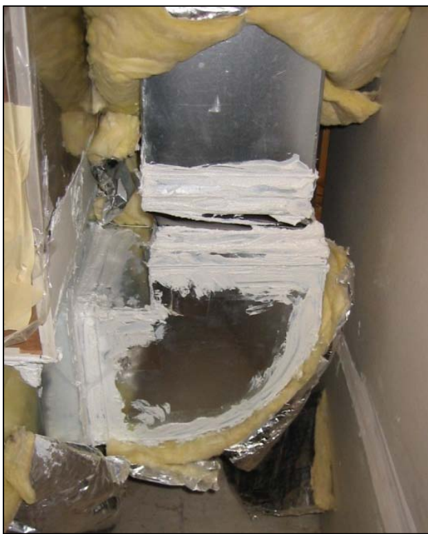
Figure 27. Duct sealers here were faced with a tight space and existing insulation. The insulation was cut and temporarily pulled back to seal connections within reach.
