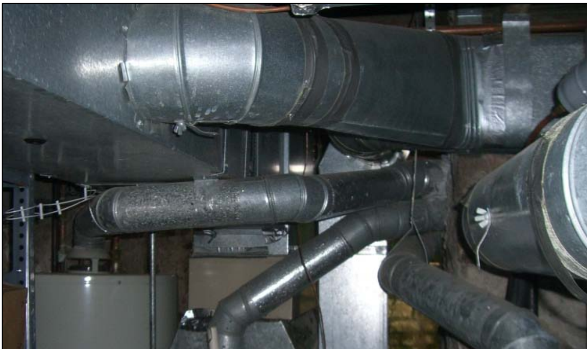
Figure 46. A tangle of metal ducts and flue pipes. Branch ducts have been sealed with duct tape which is failing (esp. in lower right). All duct seams and junctions should be sealed with mastic. Care should be taken to avoid contact with the flue piping.
