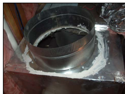
Figure 37. A branch connection collar in a sheet metal trunk. It is important to seal the collar to the trunk as well as the branch to the collar.
