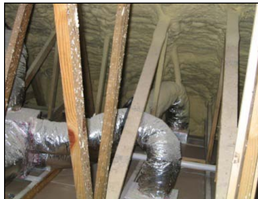
Figure 54. HVAC brought into conditioned space by applying spray foam to roof deck.
