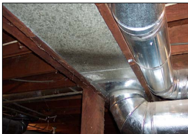
Figure 6. A “panned” return where the building cavity is used to carry air.
