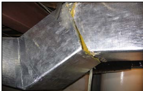
Figure 32. This duct board trunk was sealed with foil tape that has failed due to the stress put on the duct. Neither mastic nor tapes can replace proper mechanical fastening and support.
