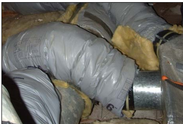
Figure 38. The inner lining of these flex duct branches have been attached to the collars, but they have not been sealed
