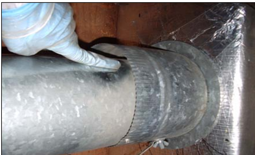
Figure 43. It appears the HVAC contractor ran out of the proper sized ducts or collars for this installation
