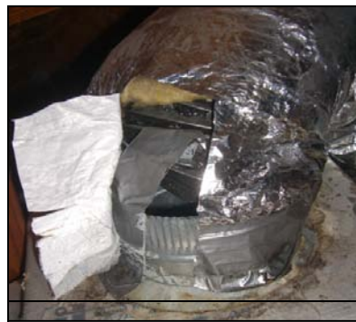
Figure 34 This flex branch never overlapped the collar and the insulation wasn't properly installed resulting in leaks and condensation.
