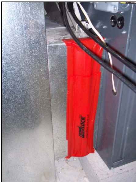
Figure 29. These polymer sheets with magnets at the edges cover the filter slot in an air conditioning system. Covers such as these can reduce leakage tremendously while allowing easy access for filter replacement.
