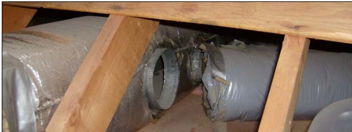
Figure 41. Disconnected ductwork resulting in conditioned air being lost to the vented attic. Homeowner was complaining of comfort issues in a secondary bedroom.
