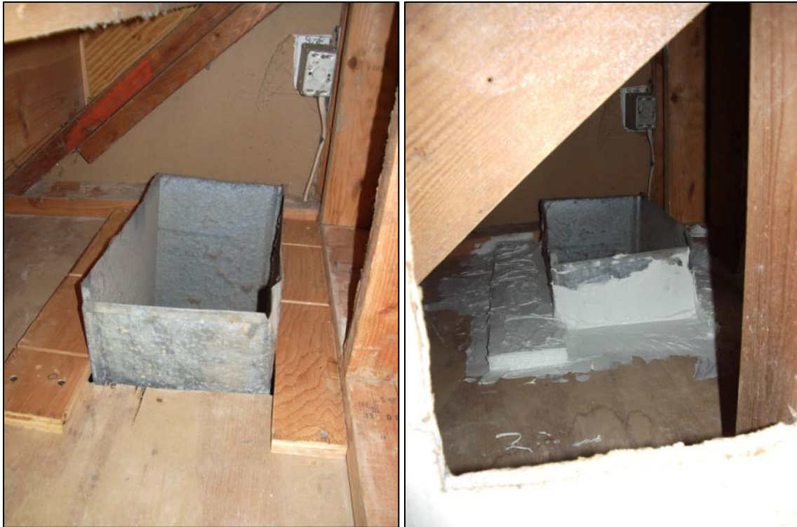
Figure 53. This space beneath a stairway was used as a return plenum. Installing a ducted return – the preferred solution – was not in the scope for this project. System performance was improved by sealing this building cavity.
