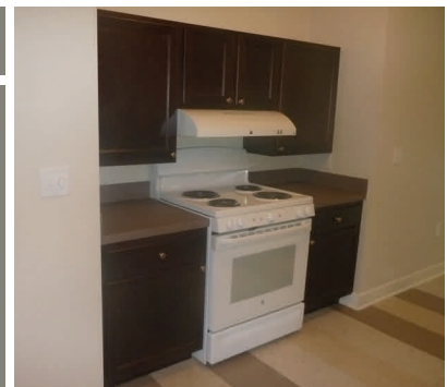
Accessible Wall Cabinets must be located no higher than 46 inches AFF, measured to the top surface of the lowest shelf.
