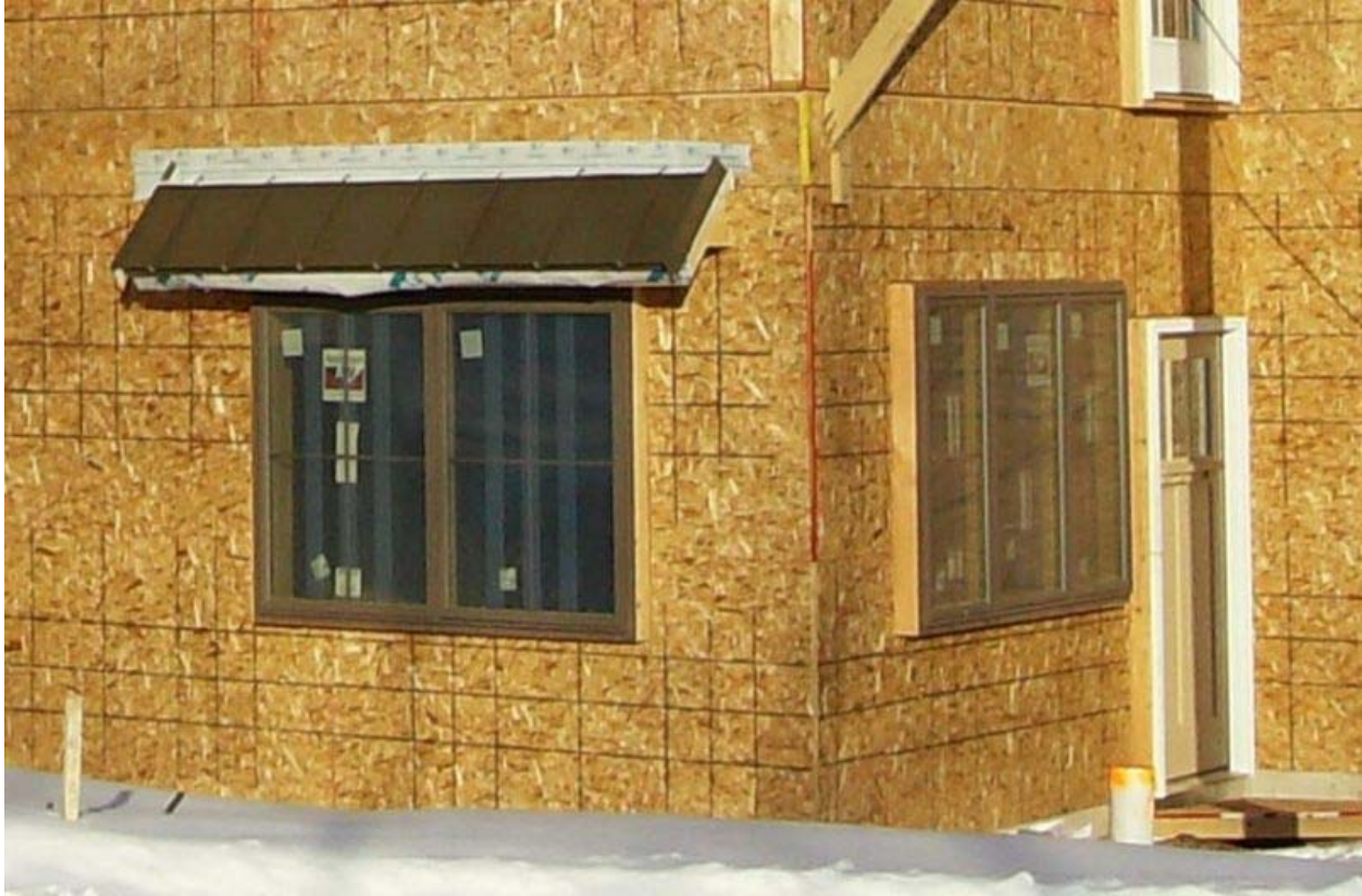
Figure 7. Outset window installation.
