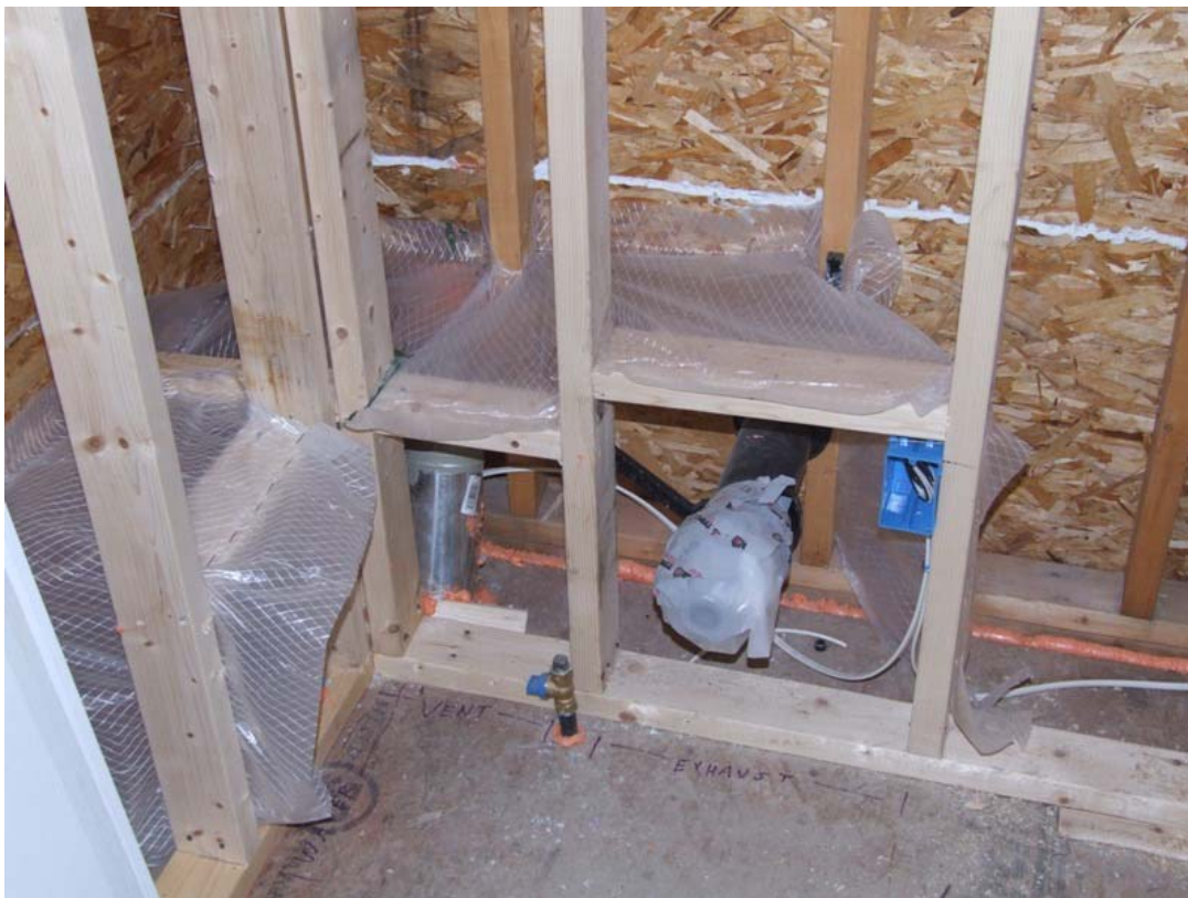
Figure 4. Insulation netting surrounds vents and plumbing penetrations in an exterior double wall. If these vents and pipes need to be accessed in the future, blown insulation in the rest of the wall need not be compromised.
