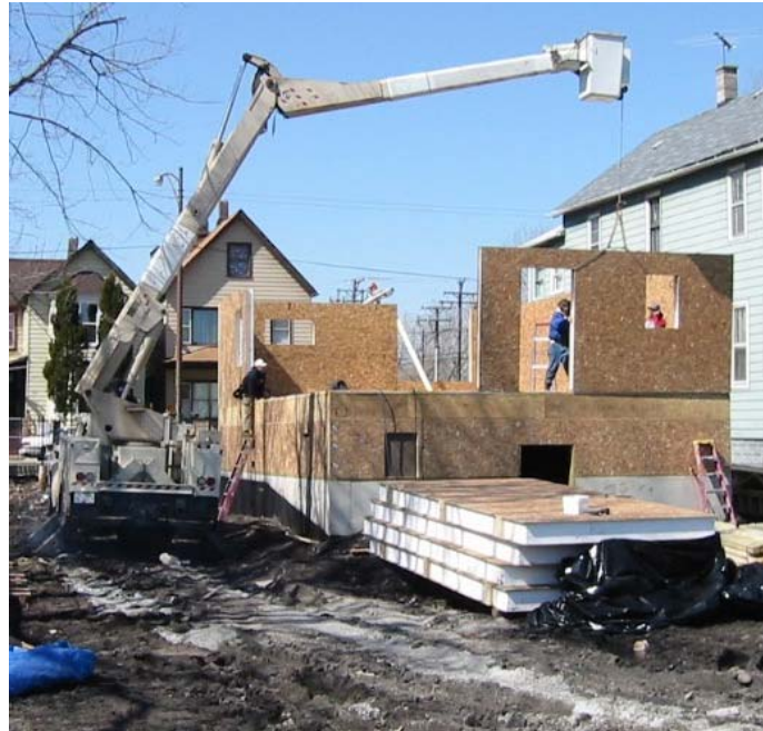
Figure 14. Wall SIPs being set on a small home.
