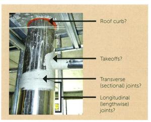
Duct leakage can be especially problematic. Trade contractors need to address duct leakage for both central and unitized ventilation. A best practice is to include specifications for duct tightness in construction documents. For example:
