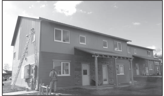
Figure 9. “With Ithaca, we’re monitoring thicker walls, 12” as compared to the prior 10”, and looking at 2 different configurations,” Lois Arena notes. Homes with R-52 wall assemblies are pursuing Passive House Certification. SWA is monitoring walls at northern and southern exposures on both homes. Photo courtesy Steven Winter Associates, Inc.
