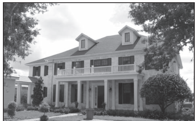
Figure 1. Building America Retrofit Alliance (BARA) and the Consortium for Advanced Residential Buildings (CARB) undertook a deep energy retrofit on a large 1995 builder spec home in Florida, to see whether 50% energy savings could be achieved both cost effectively and unobtrusively. We revisit two specific systems to check on their performance. Photo courtesy Steven Winter Associates, Inc.
