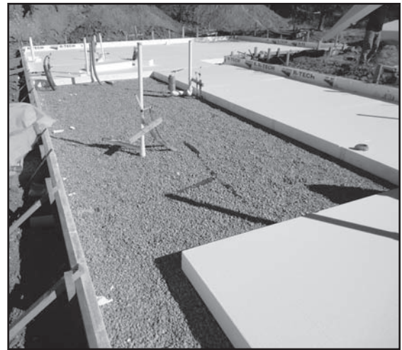
Figure 5. Insulation at slab. Image courtesy Mojarrab Stanford Architects (MoSA).
