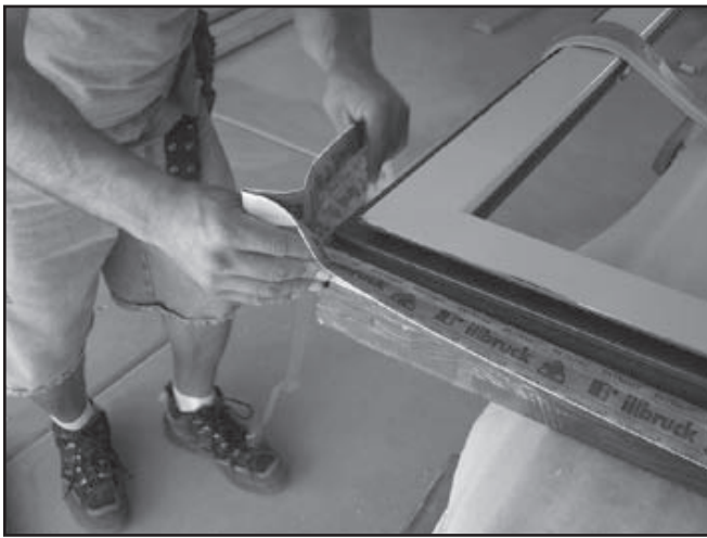
Figure 13a and 13b. Corner treatment: Illbruck Duo tape shown. Image courtesy Zola Windows.
