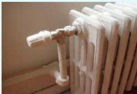
Figure 5: Two-Pipe Steam Thermostatic Radiator Valve (TRV)
