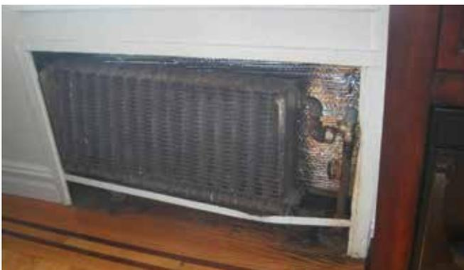
**Figure 8: Radiant barrier installed**
