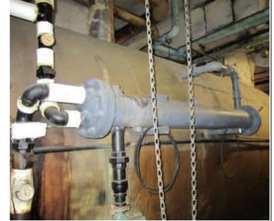
In the boiler room, most things are warm, but some really stand out. For example, boilers that burn #6 heavy oil must heat it continuously so that it flows easily. A heat exchanger (pictured above right) on the side of a boiler is a very common way of accomplishing this task, using hot water from the boiler and oil circulated between the heat exchanger and the storage tank.
